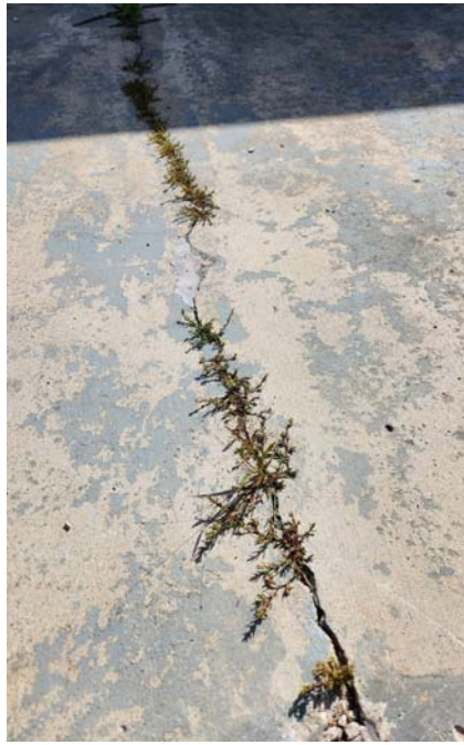
Image 45: Pool deck crack
