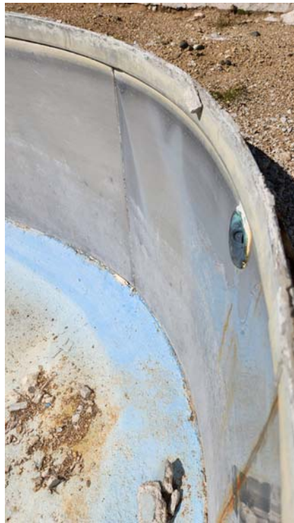
Image 47: view looking straight down showing damage to top of stainless-steel pool wall.
