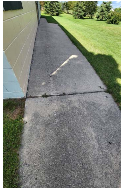
Image 17: Existing accessible path to pool entry showing cracking. Note: current path does not meet approved ramping from street parking to accessible sidewalk. Image 18: Existing sidewalk showing control joint transition along accessible route.
