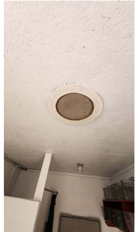
Image 7: Women's Interior Toilet View Minor cracking on wall and curtain as door Image 8: Women's Interior Ceiling View showing painted chip board and sealed vent/light well with plastic.
