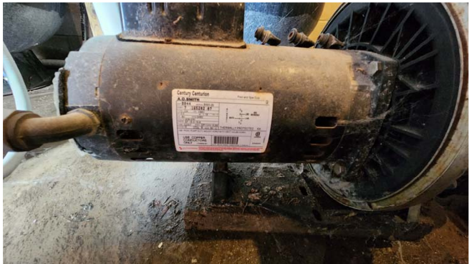
Image 58: View of one of the many pool pumps.
