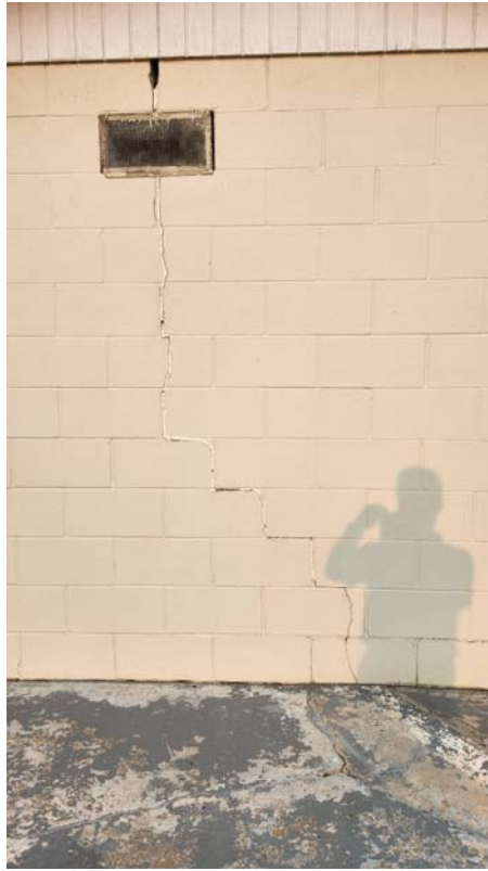
Image 13: South exterior wall of pool mechanical room showing masonry cracking due to differential shifting of the wall as there are two different substrates the current wall sits on.
