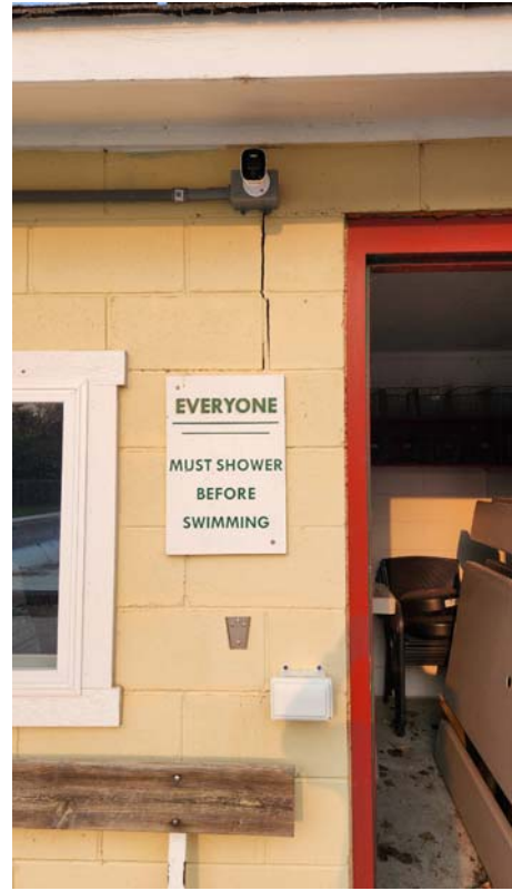
Image 13: South exterior wall of pool mechanical room showing masonry cracking due to differential shifting of the wall as there are two different substrates the current wall sits on.
