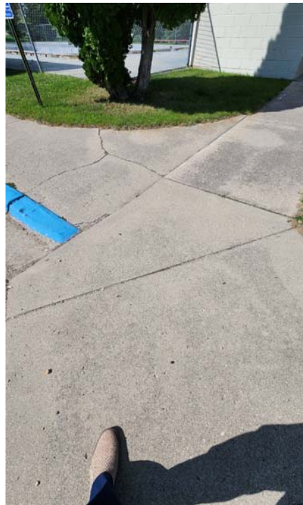
Image 17: Existing accessible path to pool entry showing cracking. Note: current path does not meet approved ramping from street parking to accessible sidewalk. Image 18: Existing sidewalk showing control joint transition along accessible route.
