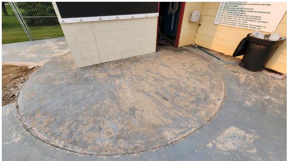
Image 15: Exterior view of Pool House showing the west addition sitting on top of The old kiddie pool resulting in differential movement of the building shell which in turn has caused the masonry wall to crack. Refer to image 13.
